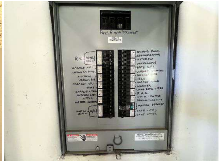
Garage sub panel breakers were labeled
