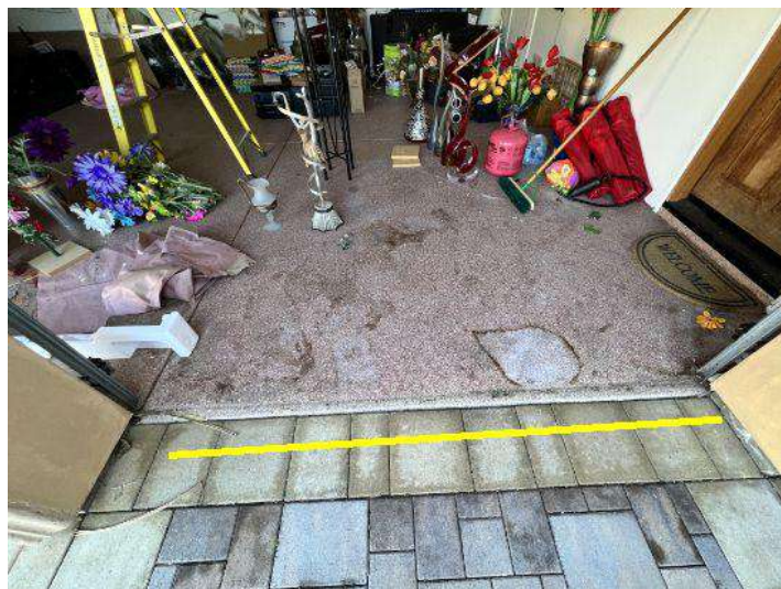
Evidence of water infiltration on the main garage floor
