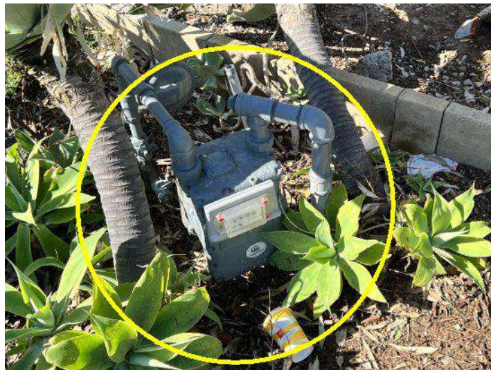
The gas meter was missing a seismic shut off valve
