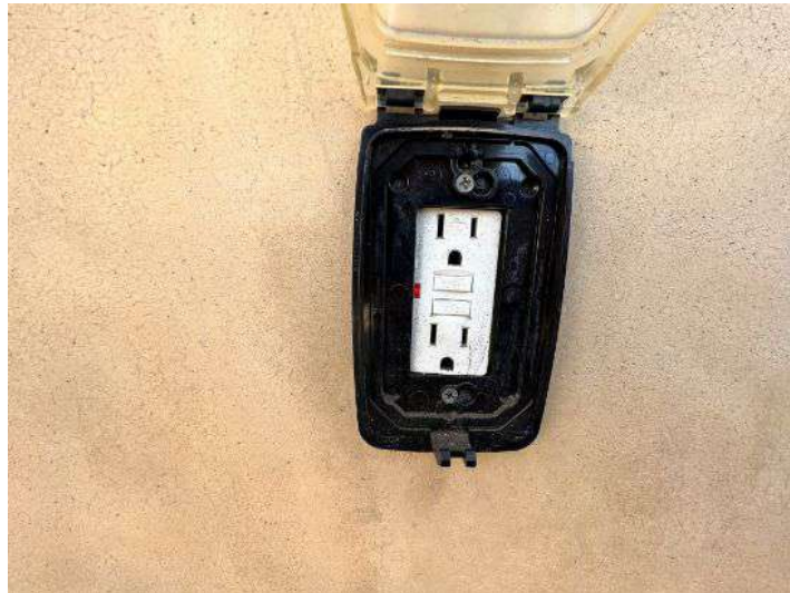
This exterior electrical receptacle was defective
