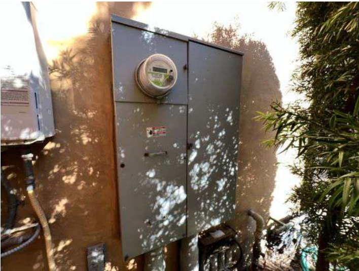
Primary electrical service disconnect near the guest house entry
