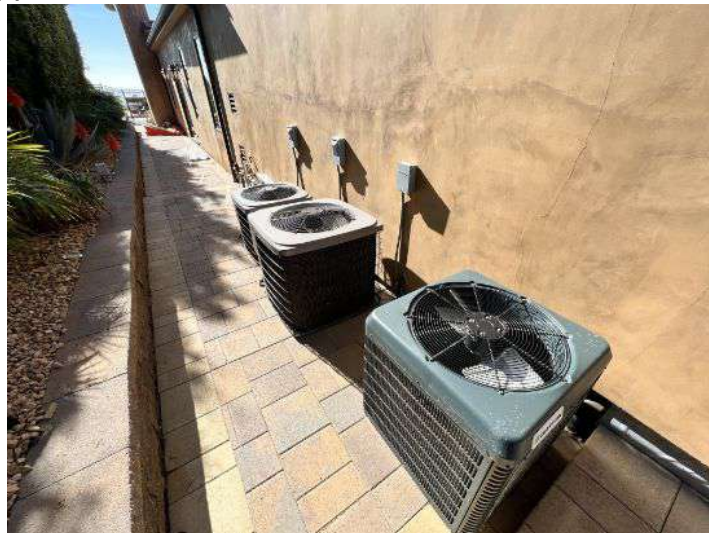
The three A/C units should be strapped down for safety
