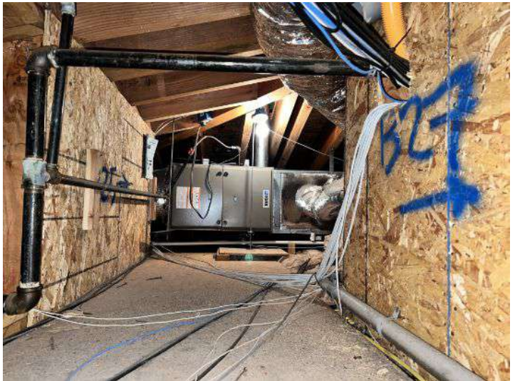
Forced air unit located above the laundry room
