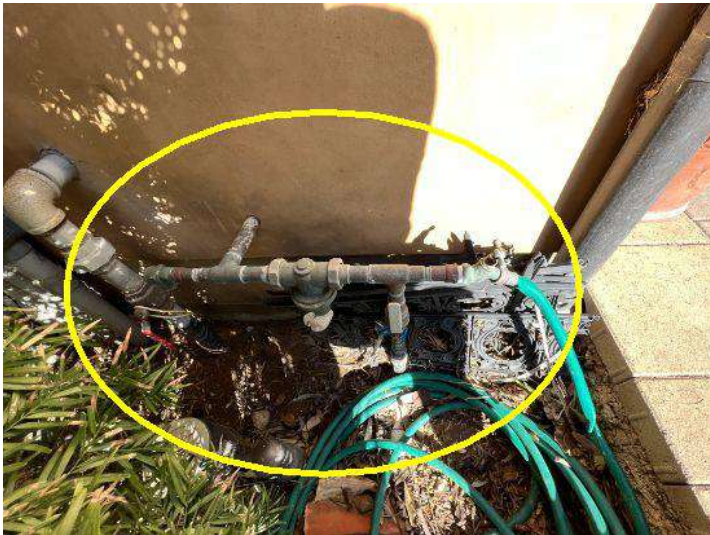
Guest house water shut off and pressure regulator shown here
