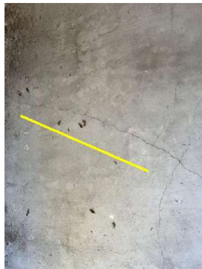
Some hairline cracks on the concrete garage floor
