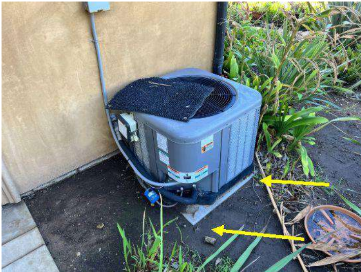
The guest house A/C unit should be raised off the ground and strapped to the base
