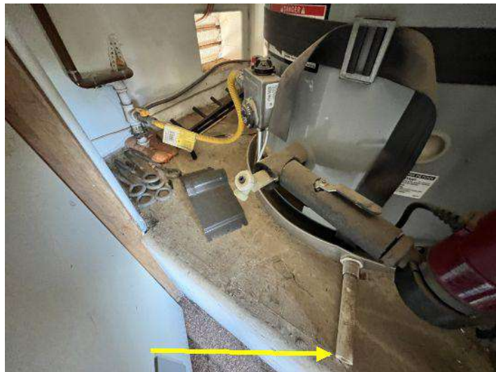
A drain pan extension pipe is recommended
