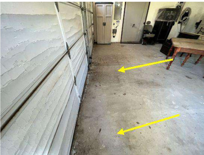
Evidence of water infiltration
