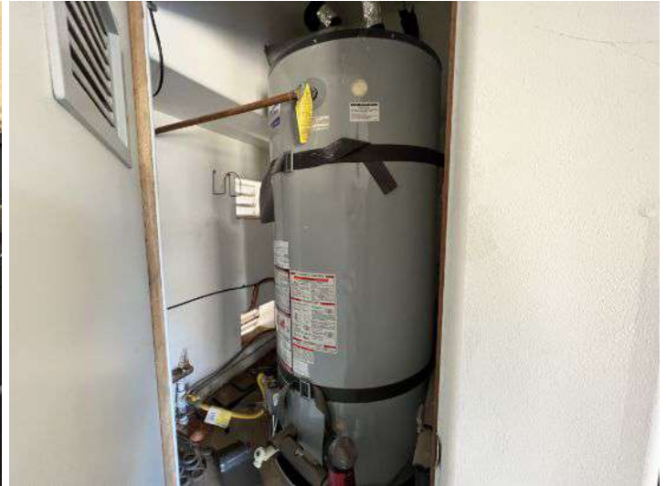
75 gallon water heater located in the garage closet
