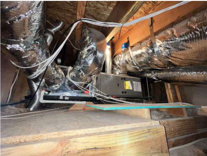
Forced air unit above the master closet
