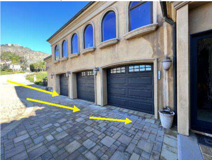
No visible drains near the main house garage doors
