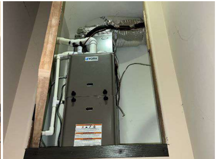
Forced air unit above the staircase
