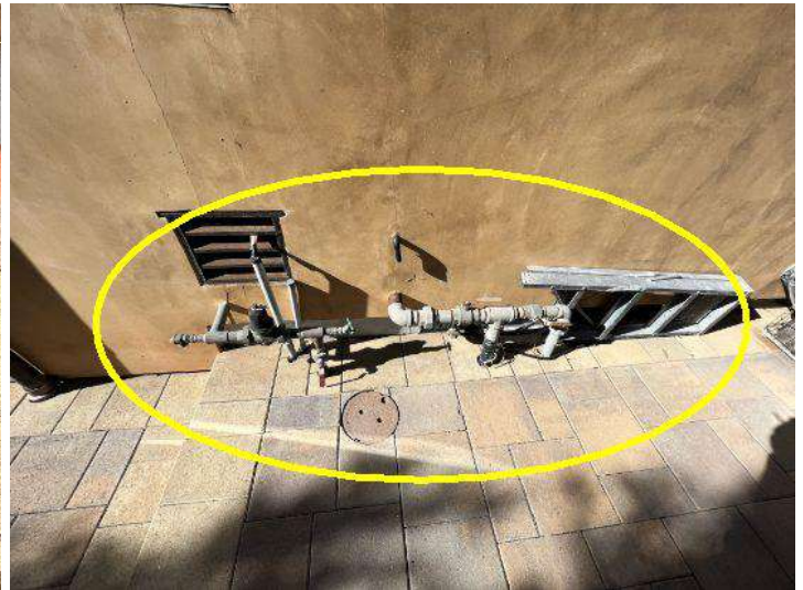
Guest house water shut off and pressure regulator shown here
