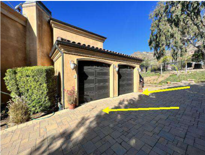
Water may drain toward the garage doors
