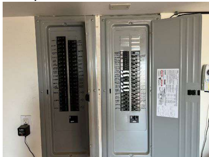
200 and 150 amp electrical sub panels located in the main house garage
