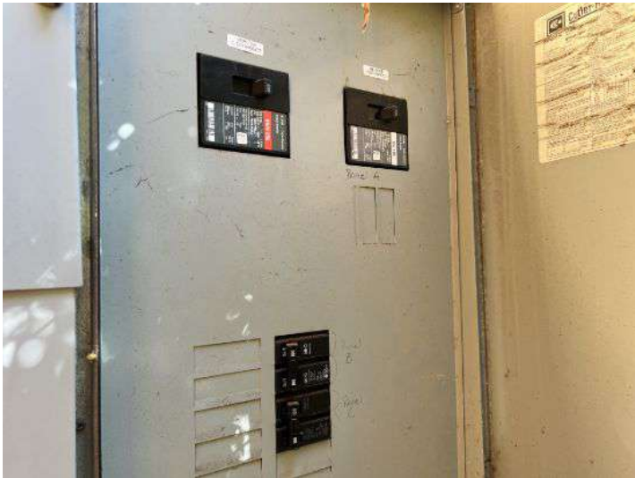
Service disconnect breakers
