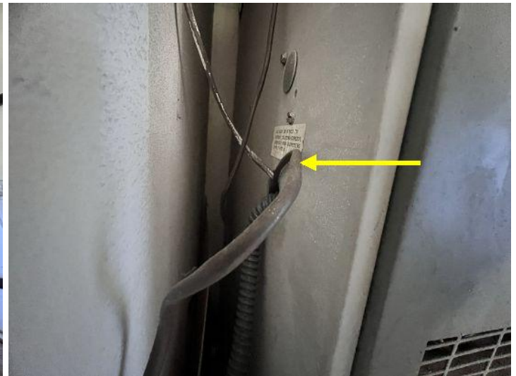
Rigid gas fitting recommended here
