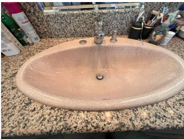
Defective sink stopper
