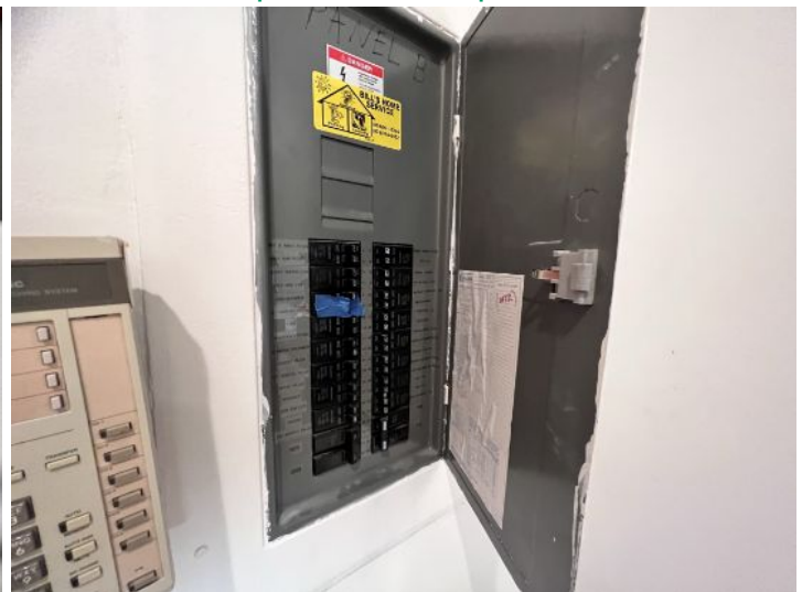
Electrical sub panel in the laundry room
