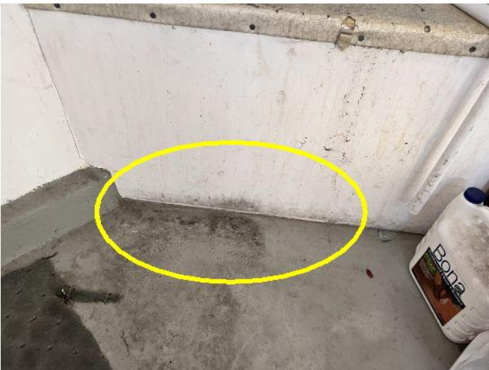
Microbial growth on the water heater base
