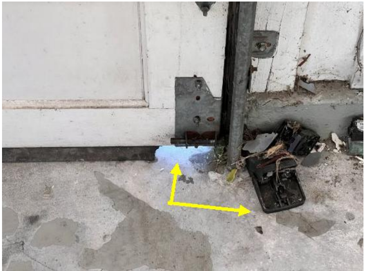
Damaged weatherstripping and detached sensor shown here
