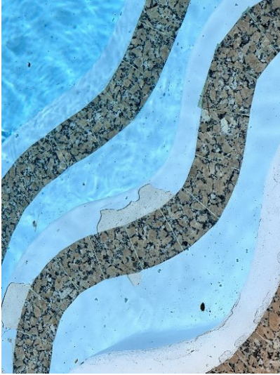
Chipped plaster on the pool steps
