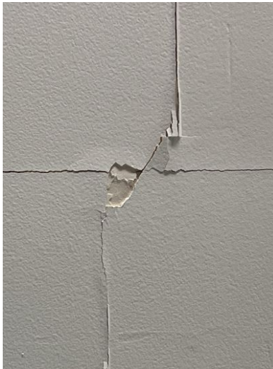
Cracks on the garage ceiling
