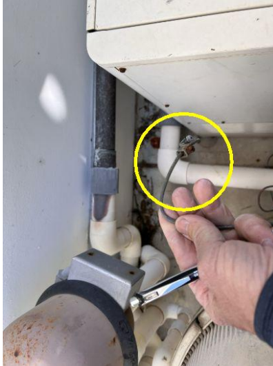
Disconnected electrical ground wires at the pool equipment
