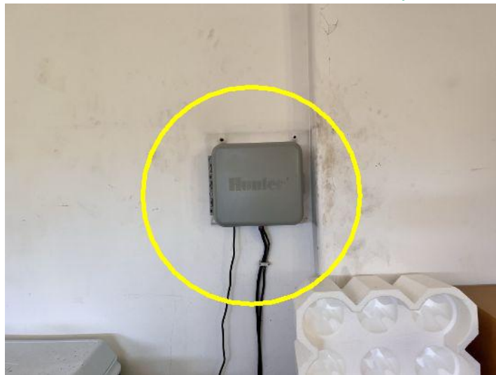
Landscape sprinkler timer box located in the garage
