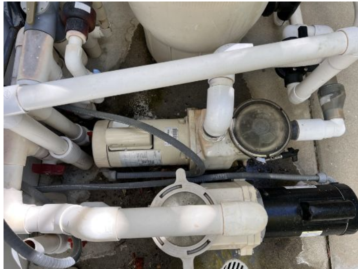
One pump appeared to be leaking
