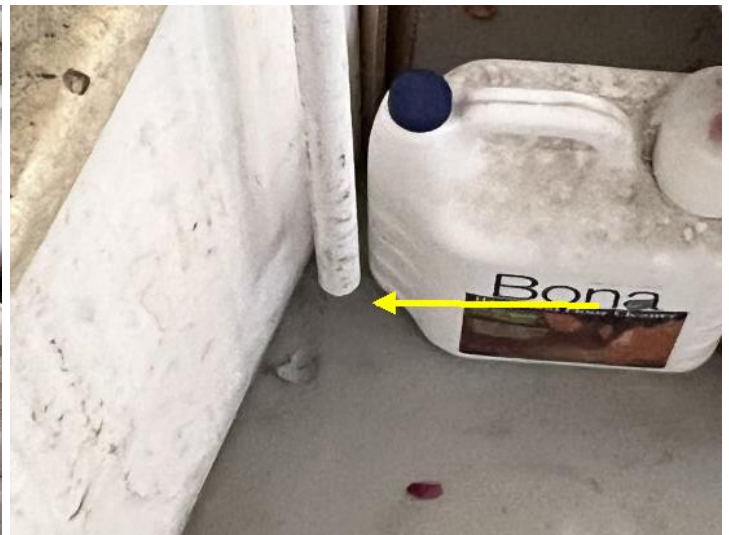
A drain pan extension pipe is recommended
