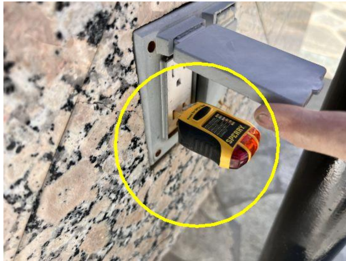
Defective receptacle on the outdoor kitchen island
