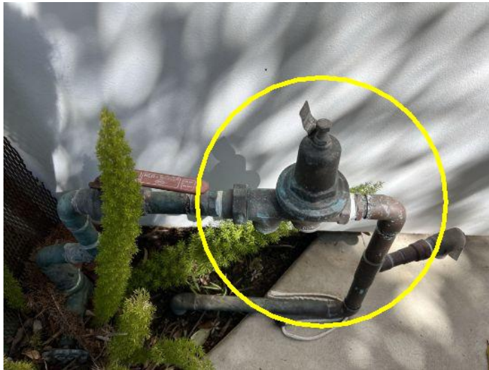
Water pressure regulator and water shut off on the right side of the house
