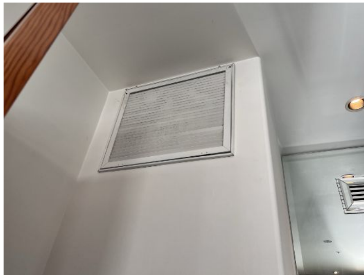
Air returns and filters were dirty
