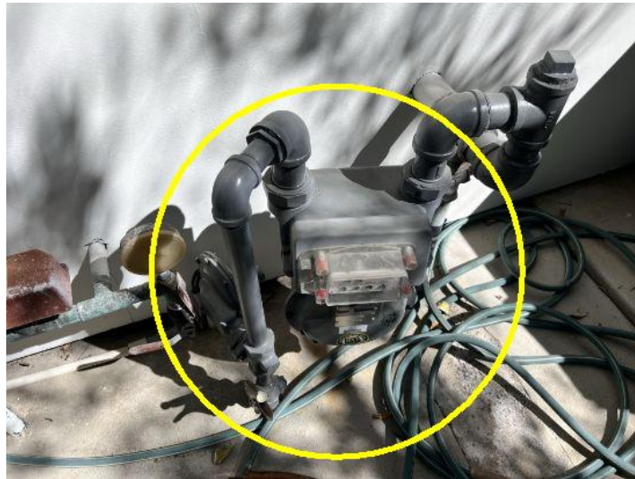
Gas meter and shut off valve on the right side of the house
