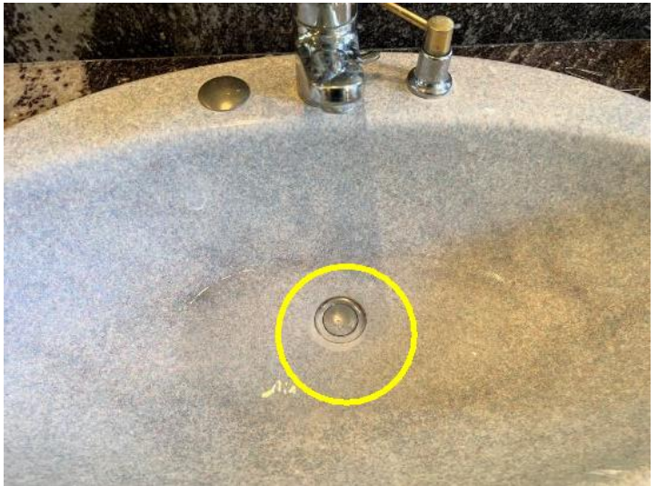
Defective master sink stopper
