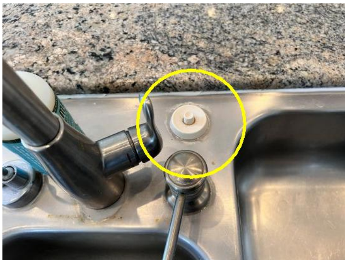
This garbage disposal did not operate when tested
