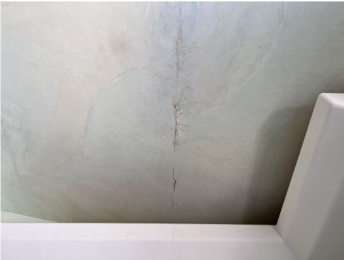
Evidence of water damage on the master bedroom ceiling
