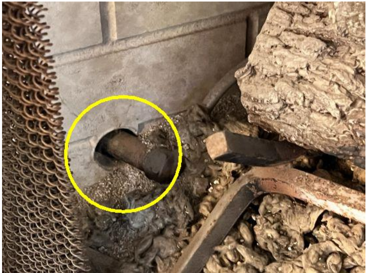
This gap should be sealed for safety
