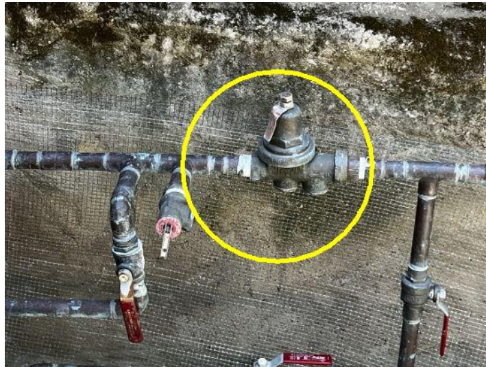
Water pressure regulator shown here
