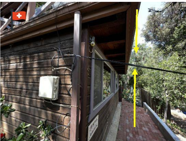
This low voltage wire was across the walkway
