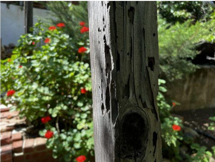
Termite damaged patio cover
