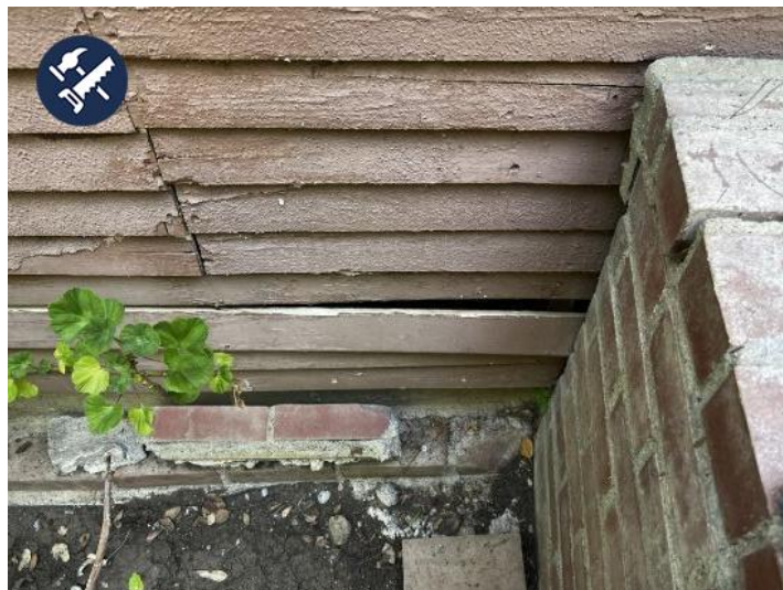
Damaged wood siding in some areas
