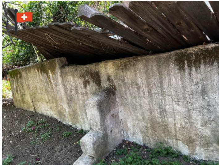
Leaning concrete wall behind the property
