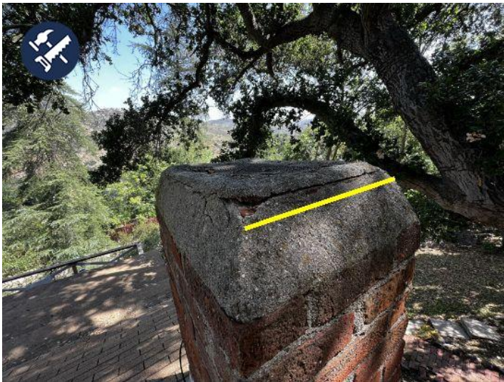
Cracked mortar
