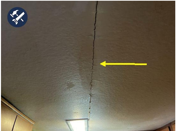
Cracked acoustical ceiling
