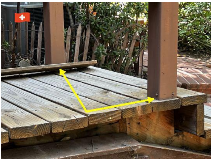
Balcony posts were not properly supported
