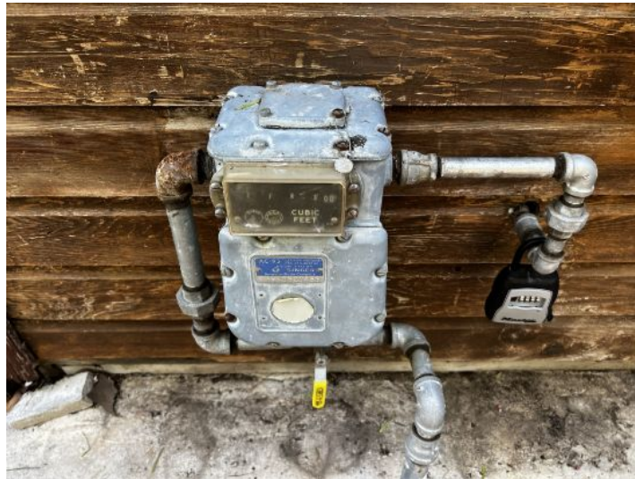
Gas meter and shut off valve shown here
