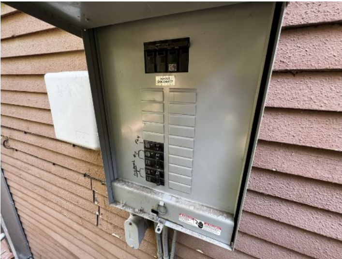
Newer electrical panel had been installed for the HVAC system
