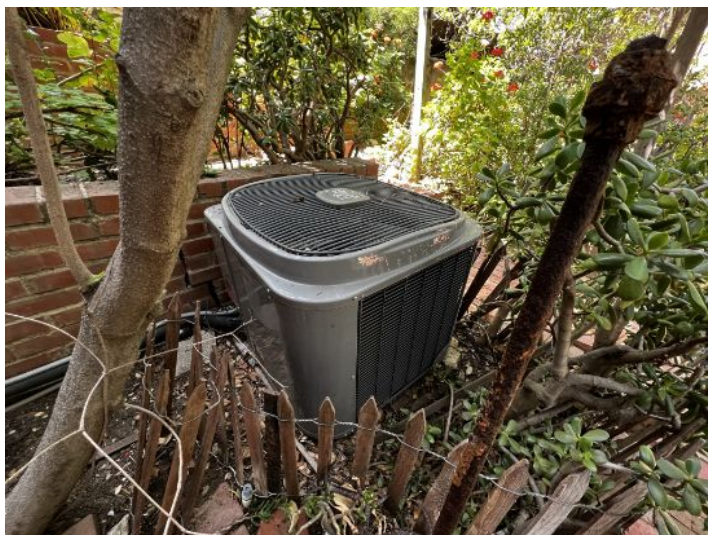
Newer A/C unit should be level
