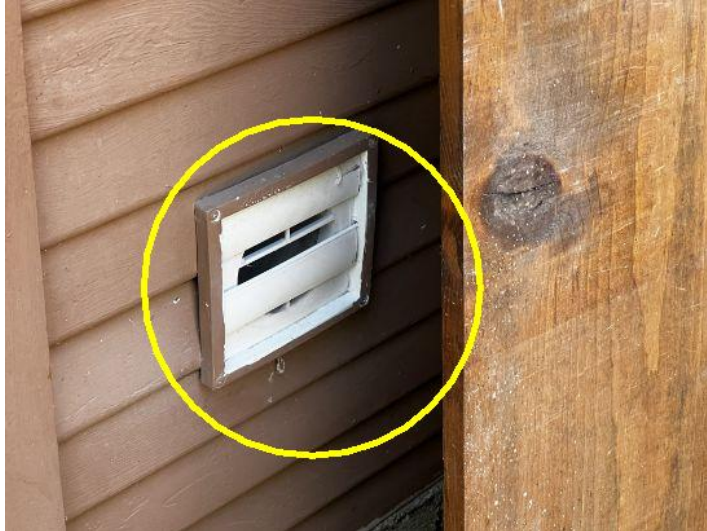
Damaged dryer vent
