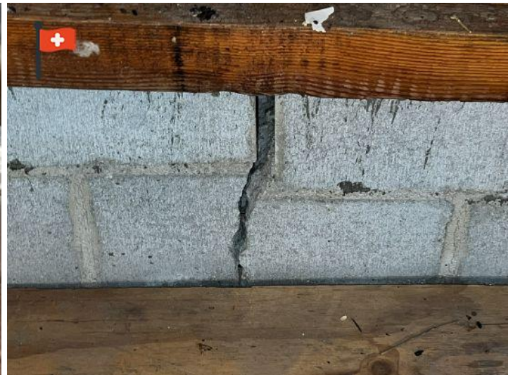
Foundation wall crack
