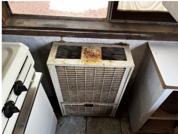
This kitchen wall heater should be removed for safety
