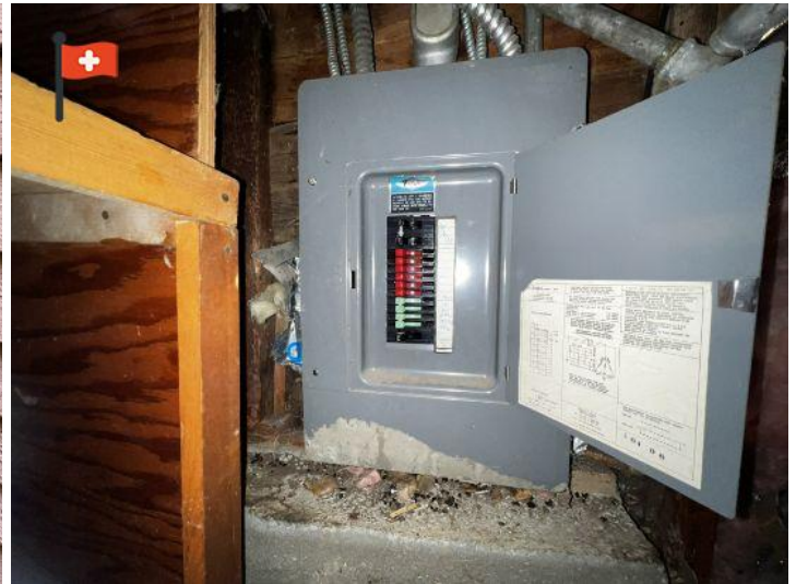
Zinsco electrical panel shown here
