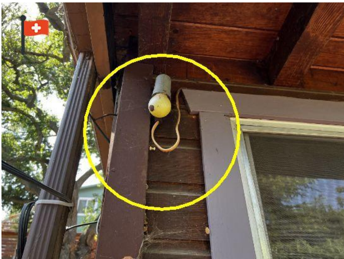
Exterior light fixtures were not intalled properly
