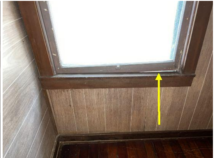
Windows were out of alignment, possibly caused by shifting foundation
